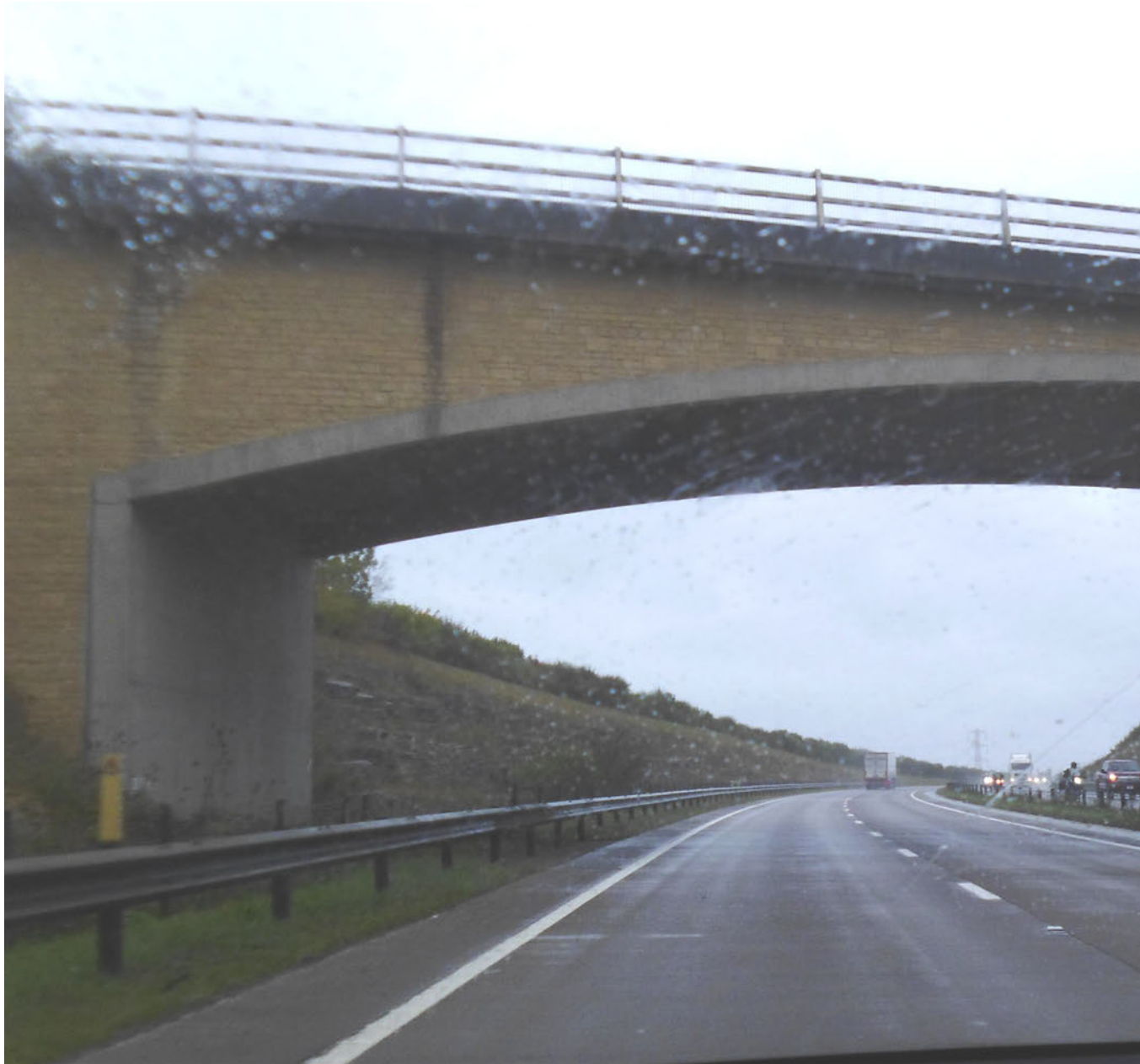
Pic.3 Option 12 would widen the existing A417, a boundary of Stockwell Farm in both directions, in part using wide verges left for the purpose c25 years ago and owned by Glos.CC, taking a small amount of extra land but leaving the farm and all wildlife intact, thus saving the massive cost of Compulsory Purchase and 2 over bridges
